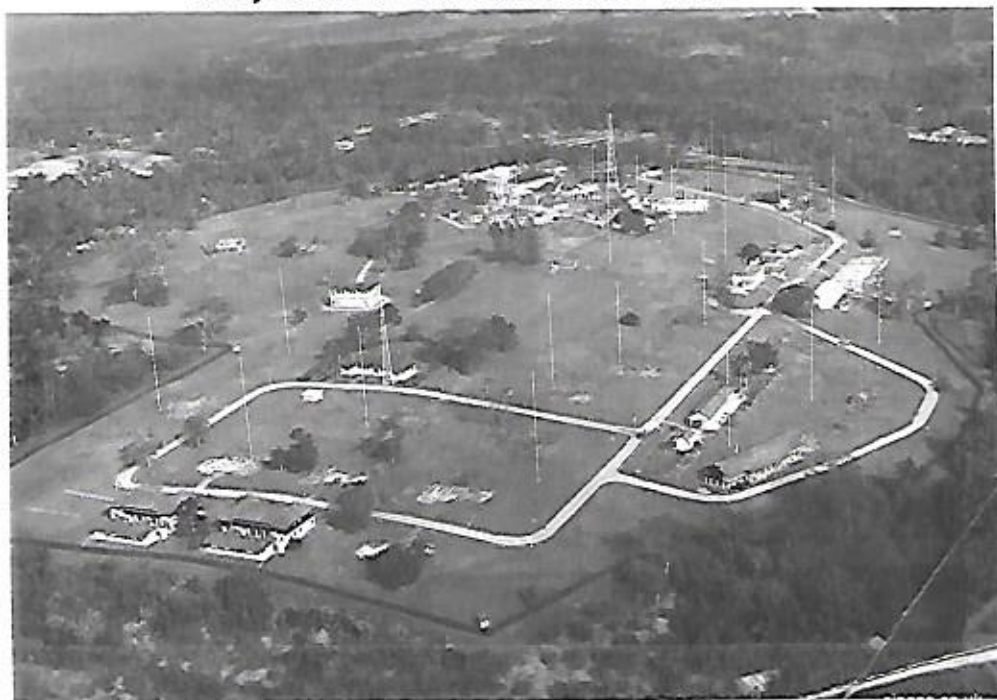
Kranji Wireless Transmitter Station - 1939
