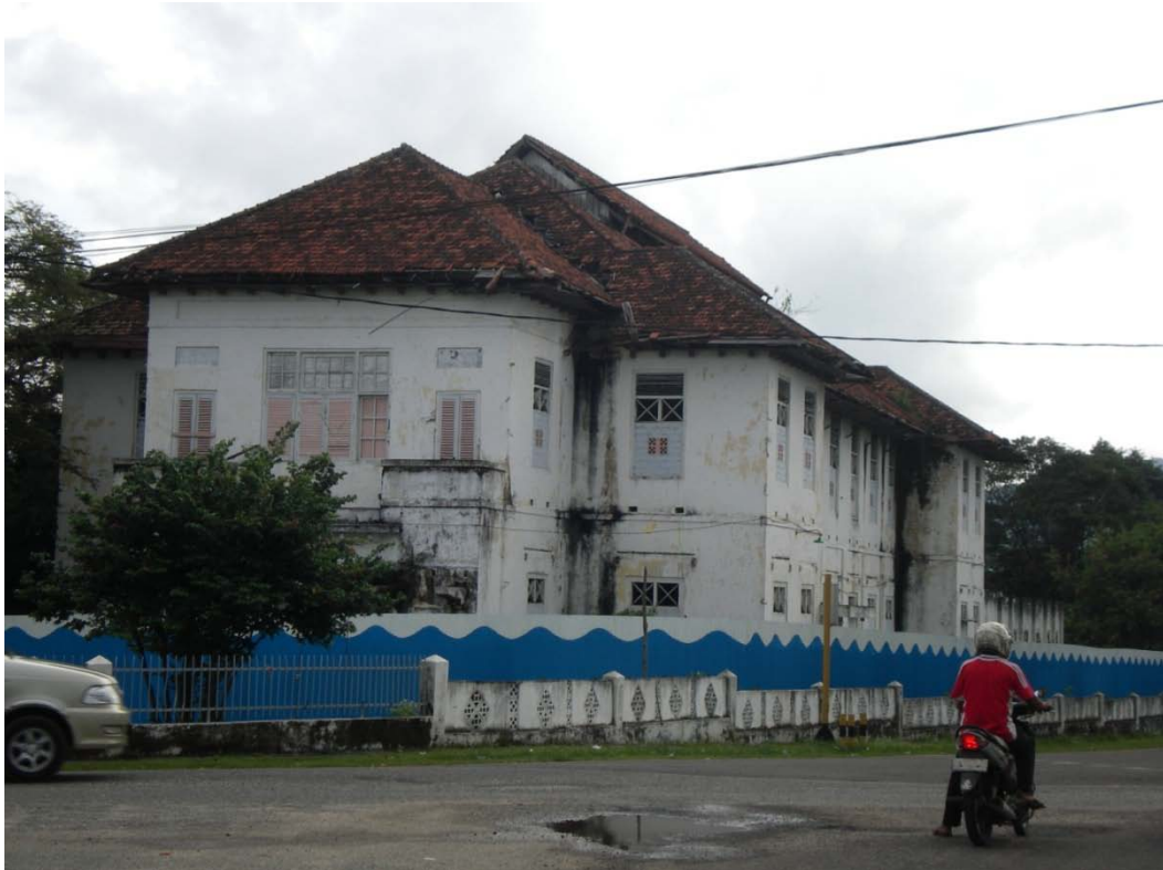
The Tinwinning Building
